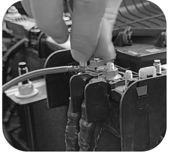
Install the power terminal to the battery.
