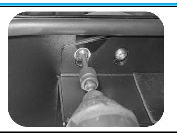
Bolt the rear feet of the sports bar to the Load-Lid through the face plate, using the following fasteners:
