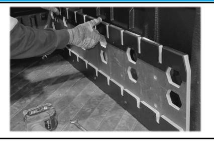
Position the side boards in place. Make sure to have the rough side facing out. The boards will be labelled with left (L) and right (R) cutouts
