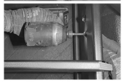
Now with the sides correctly distanced, tighten all the loose bolts
