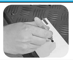
Mark all holes through the template onto the Load-Lid.
