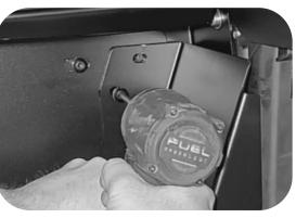
Install the corner bracket to cover the open area in the front corners.
