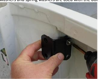
Step 7) Install the rear top bracket (PRT-004210) to the base bracket, ensure steel washers and spring washers are used with the bolts.
