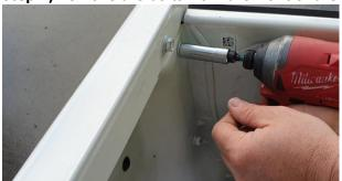
Step 5) Remove the bolts from the rear of the wellside.
