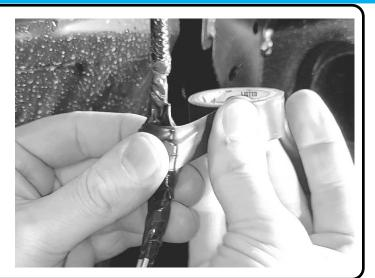
Wrap the entire section with insulation tape.
