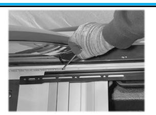
Slide the thread plates down the track and line each one up roughly with the circled positions on the base brackets.
